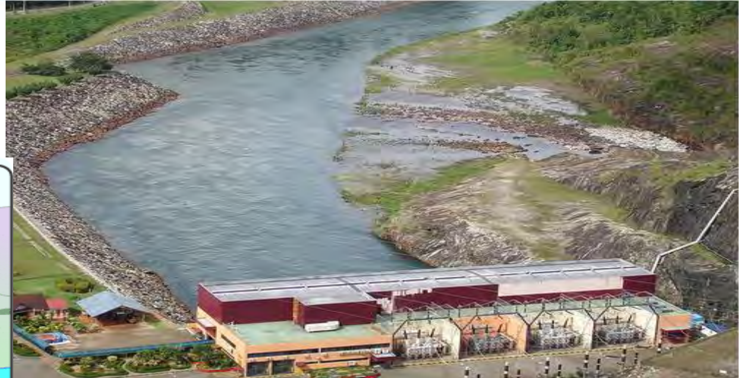
Sultan Mahmud Power Station, Kenyir
