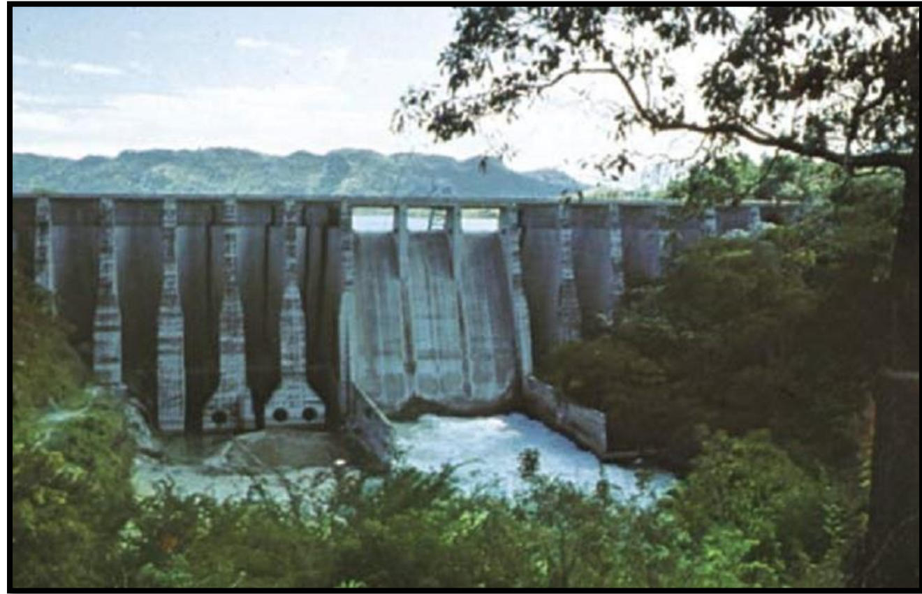
Péligre Dam, Artibonite River, Haiti
