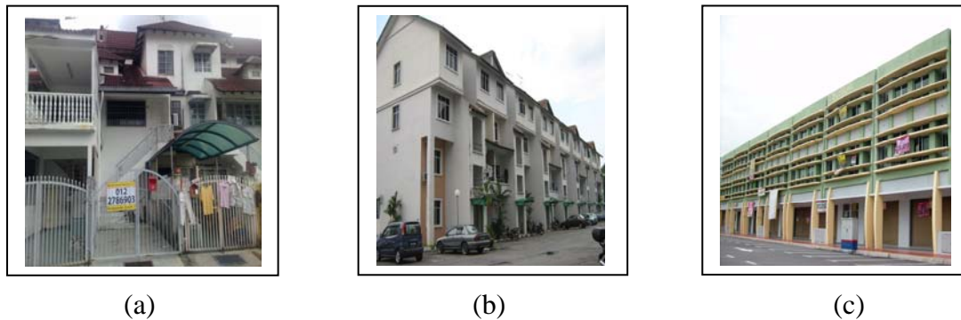
Figure 3: (a) & (b) Type of townhouse and (c) Mix shop houses at below and residential houses at above
