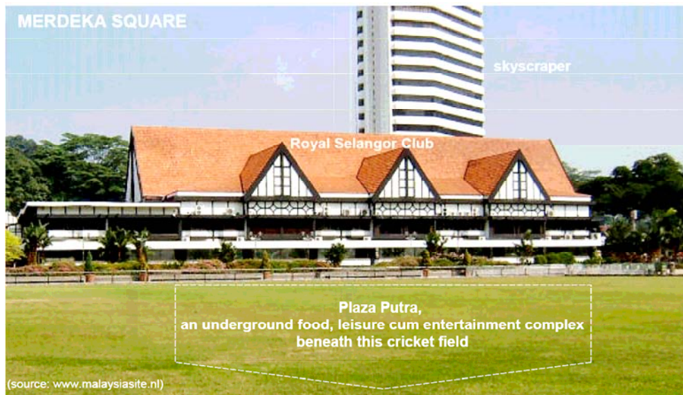
Fig. 22: Examples of modern constructions with vertical component.
